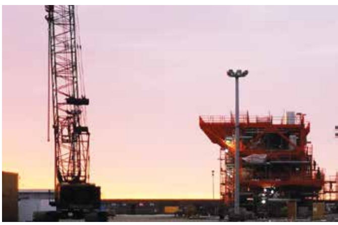
Platform currently under construction in Kazakhstan
