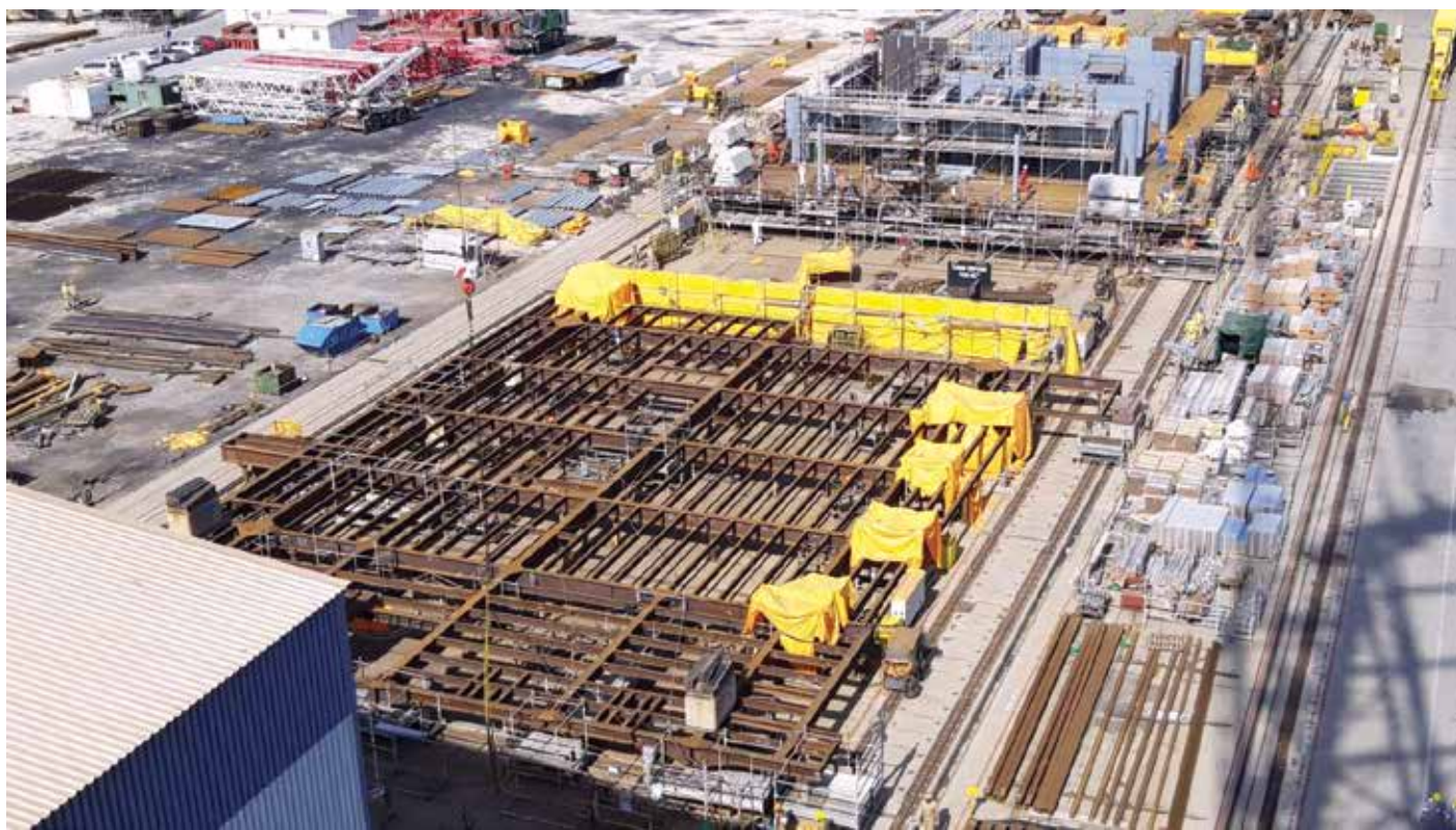
Qatar: The new living quarters structures
